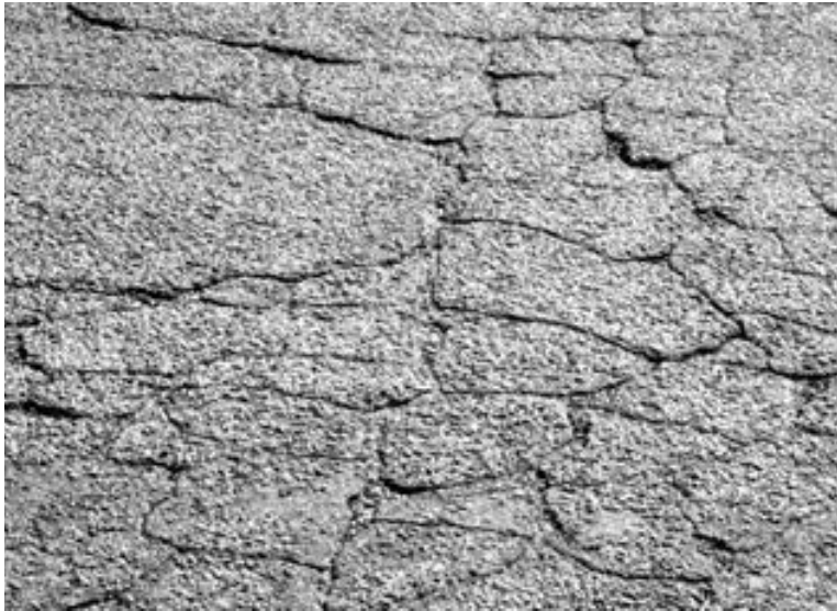
Figure 1.1 Pavement Showing Block Cracking Distress
