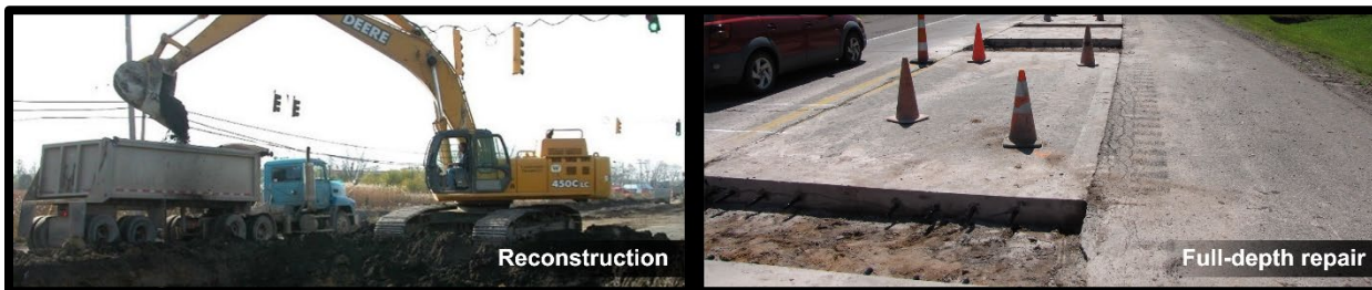
Figure 9: Examples of Reconstruction Treatments. (Left) reconstructing a road and (right) road prepared for full-depth repair.
