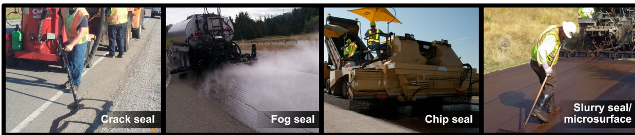
Figure 11: Examples of Capital Preventive Maintenance Treatments. (From left) crack seal, fog seal, chip seal, and slurry seal/microsurface.
