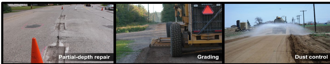
Figure 11: Examples of Capital Preventive Maintenance Treatments (continued). (From left) concrete road prepared for partial-depth repair, gravel road undergoing maintenance grading, and gravel road receiving dust control application (dust control photo courtesy of Weld County, Colorado, weldgov.com).
