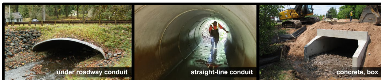
Figure C-1: Examples of Culverts. Culverts allow water to pass under the roadway (left), they are straight-line conduits with no intermediate drainage structures (middle), and they come in various materials (left: metal; middle and right: concrete) and shapes (left: arch; middle: round; right: box).
