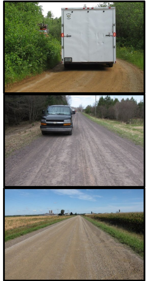
Figure 8: Road IBR Numbers. Top – Road with IBR number of 1 road that has poor surface width, poor drainage adequacy, and poor structural adequacy. Middle – Road IBR number of 7 that has fair surface width, fair drainage adequacy, and fair structural adequacy. Bottom – Road with IBR number of 9 road that has good surface width, good drainage
